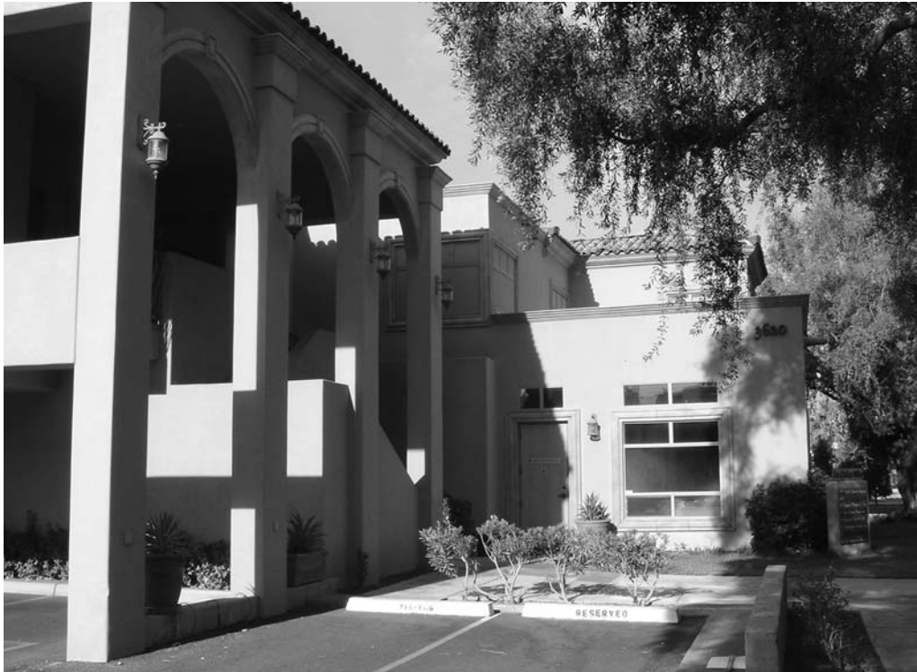
Figure 8.10 Office Building in Phoenix Where We Remodeled Suites
