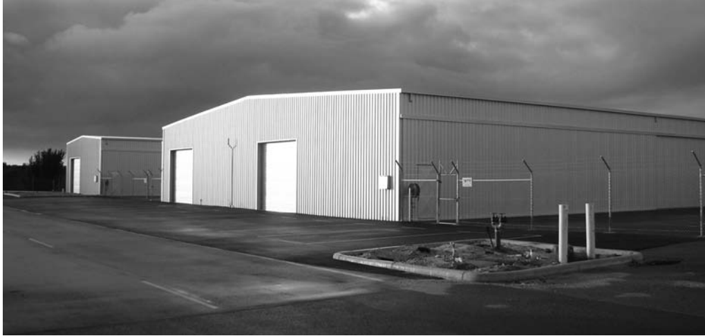
Figure 8.9 Another View of the Hangars
