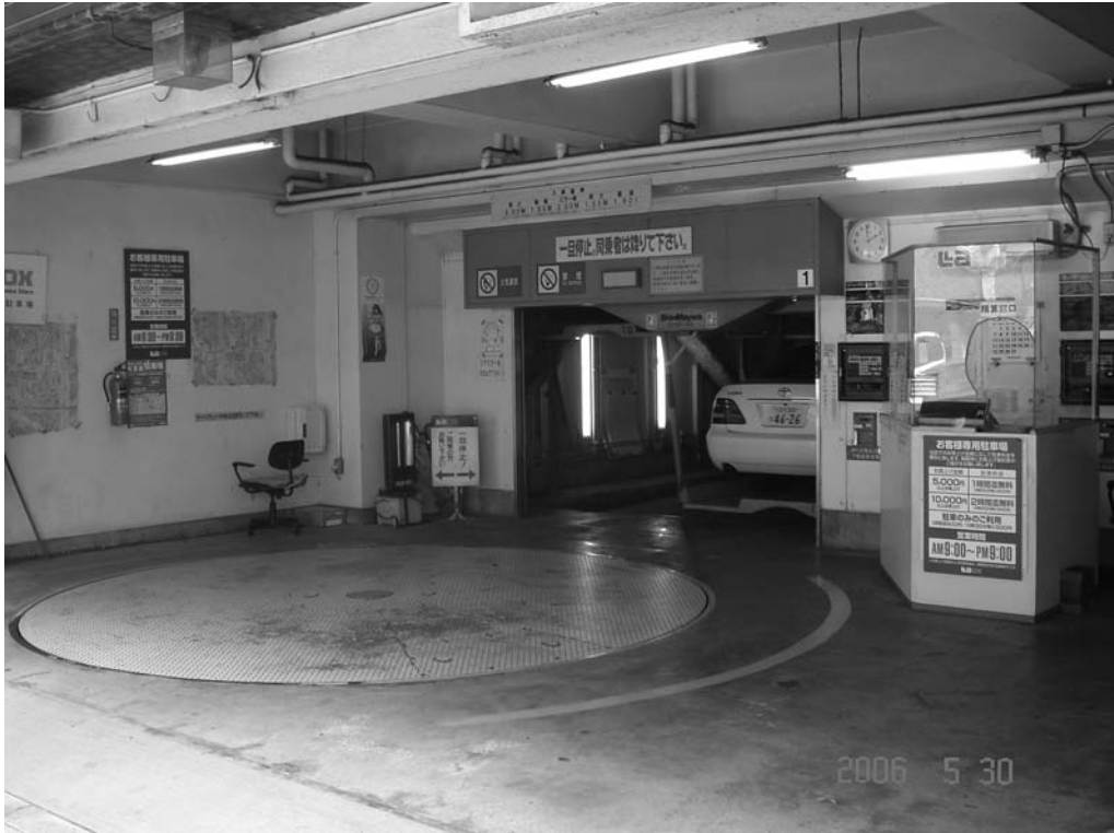
Figure 8.2 Entrance to Japanese Car-Parking System (Note the rotating platform to spin your car around when you back out).
