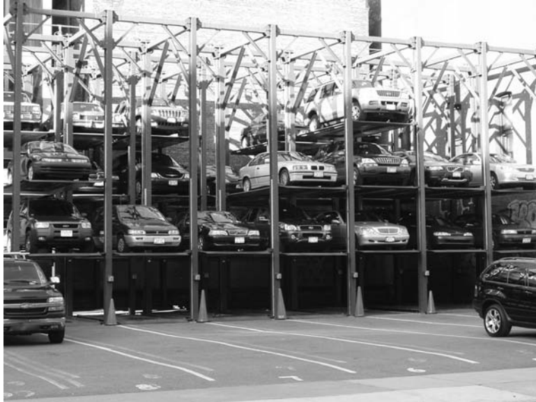
Figure 8.3 Four-Layer Stacked Parking System, New York City
