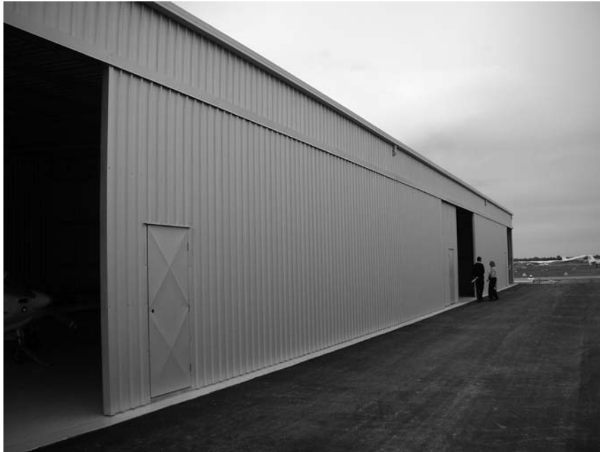
Figure 8.8 Completed Hangar with Aircraft Inside
