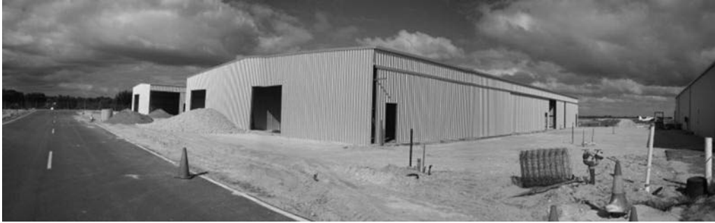
Figure 8.7 Hangars Being Constructed at Jandakot Airport near Perth
