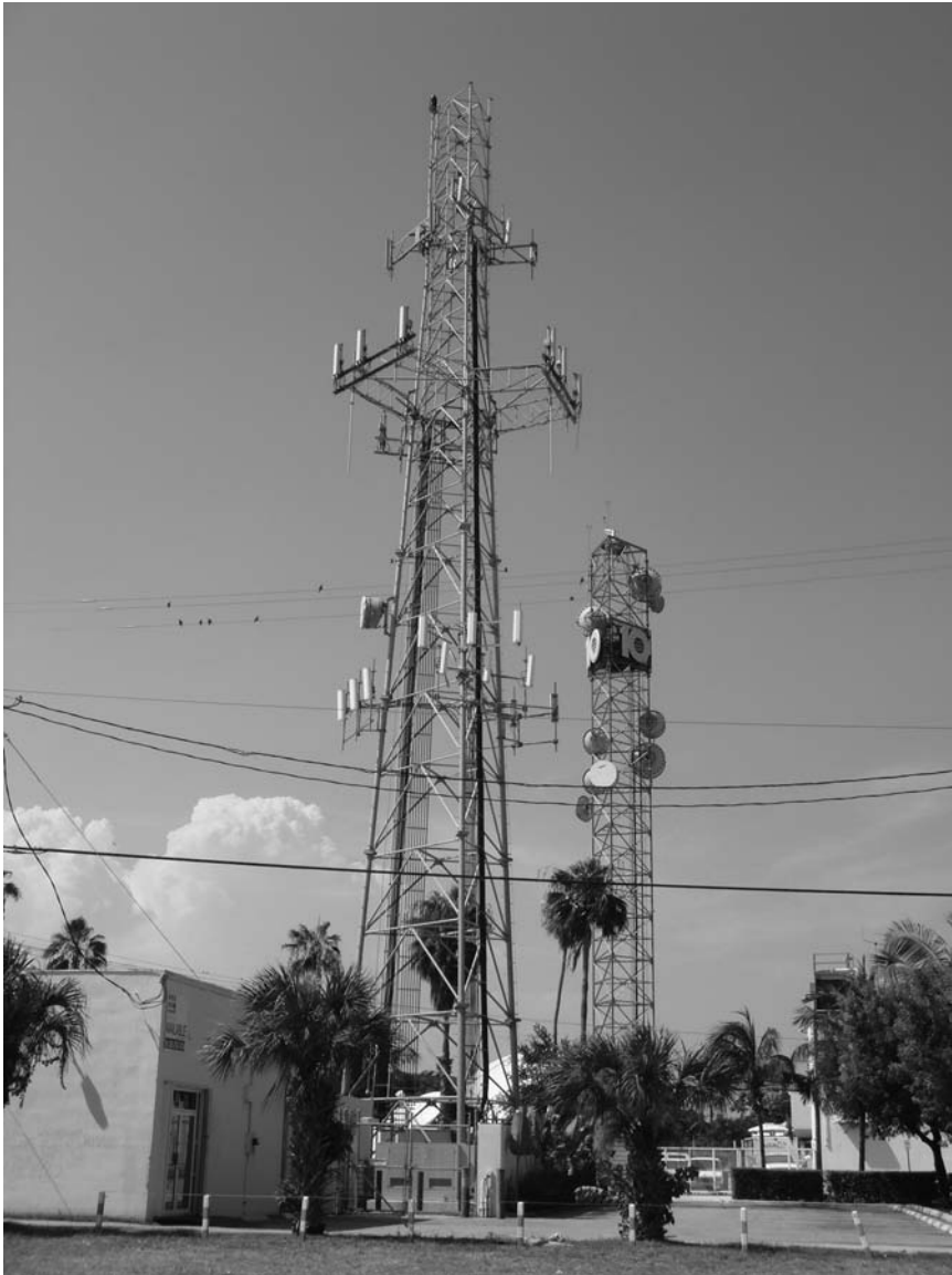
Figure 8.1 Towers with Cellular Antennas and Microwave Dishes
